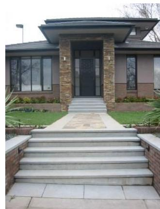
An important consideration with this type of product is the ability of the background or substrate to support the weight of the stone cladding. The
